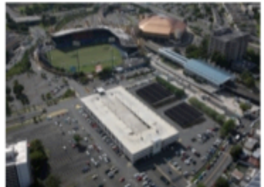
584KW PV System to be installed at the Onofre Carballeira Sports Complex in Bayamón, PR
