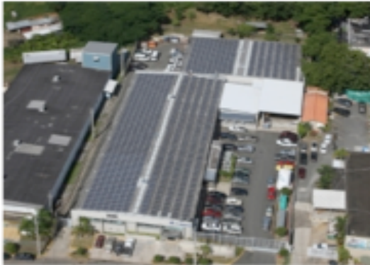
Aerial view of Aireko Enterprises' 260 KW PV System
